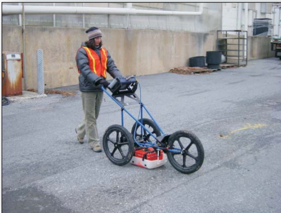
High-resolution utility mapping using UtilityScan GPR system
