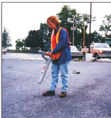
Mapping conduits with radio-frequency pipe locators
