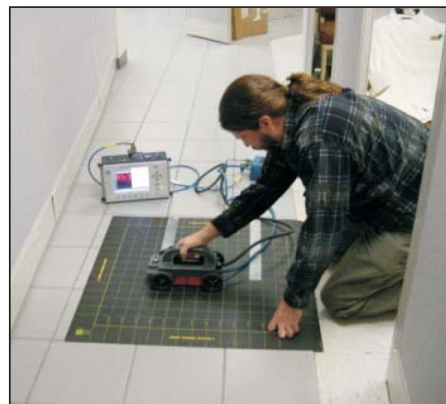
Three-dimensional GPR surveying to map embedded hazards and obstructions
